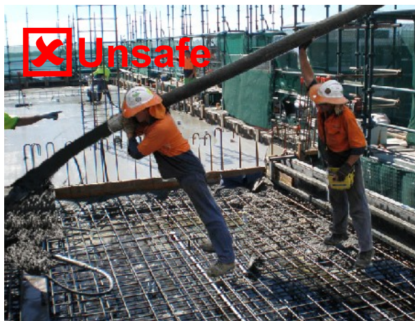
Figure 5 – Workers stretching hose for additional reach. This is an unsafe work practice.
